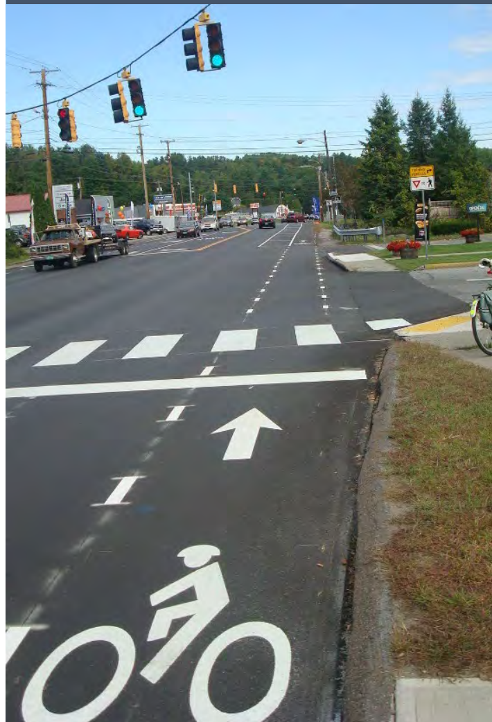
Figure 14. A standard block pattern crosswalk and bike lane pavement markings are shown as part of the Barre-Montpelier Road Diet project in Berlin.
