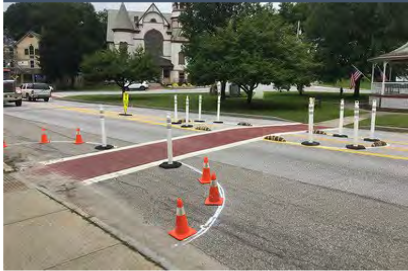
Figure 6. Demonstration shared use path and parklet along a Class 1 section of VT Route 12 in downtown Bethel, part of the Bethel Better Block initiative. To meet national standards this project would have needed to use a green paint, instead of blue, with no intermittent artwork, and added vertical delineation along the edge, in addition to the hay.
