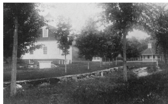
1869 view of brook walls and bottling house
